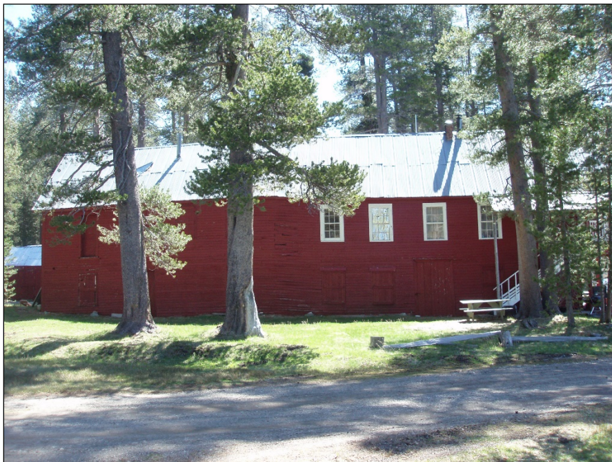
Photo 7 of 19: Webber Lake Hotel west elevation, looking east
