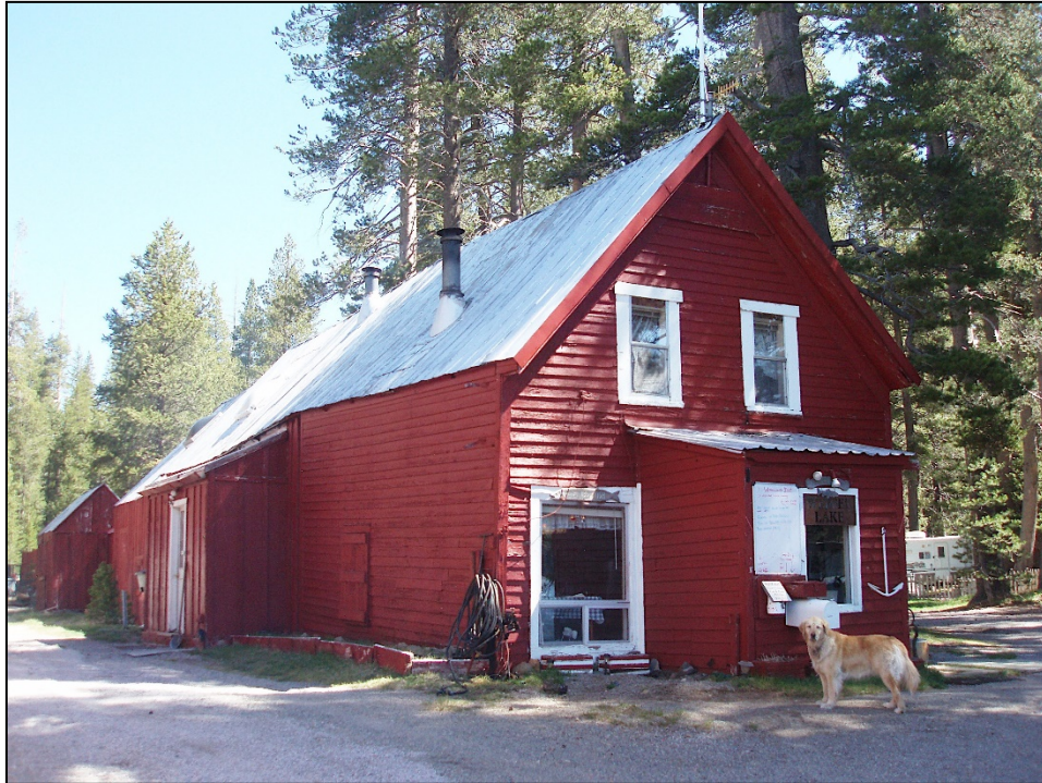
Photo 1 of 19: Webber Lake Station, south elevation, looking northeast
