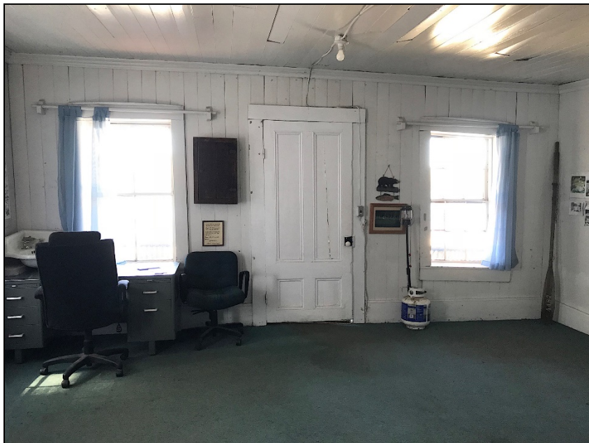
Photo 9 of 19: Webber Lake Hotel south wall in Room 101, looking south
