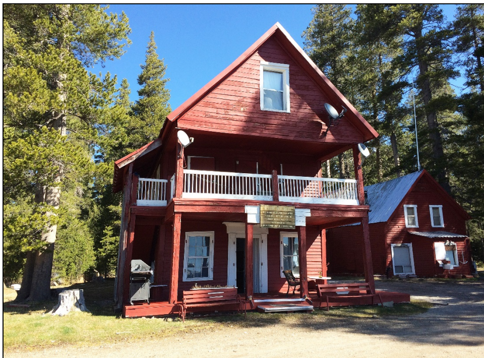
Photo 2 of 19: Webber Lake Hotel, south elevation, looking northeast
