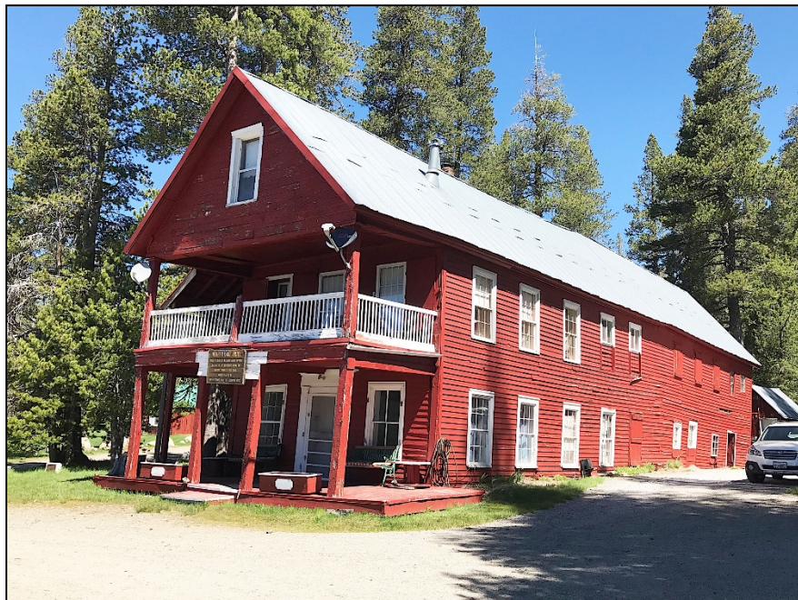
Photo 4 of 19: Webber Lake Hotel east elevation, looking northwest
